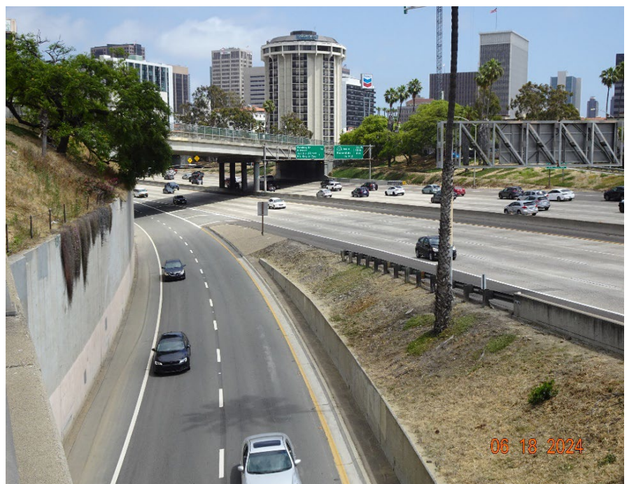
June 2024 – HyRAP® after 2 Years, approximately 24 million vehicle loadings
