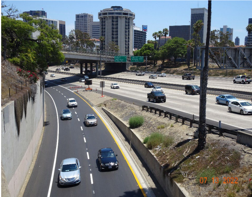
July 2022 – HyRAP® after initial placement
